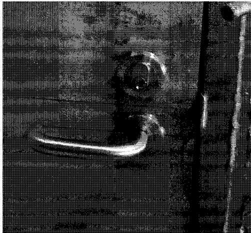
Typical installation of a 6000 Series Mortice Lockset with Novas B01/51/SSS Sprung Levers.
